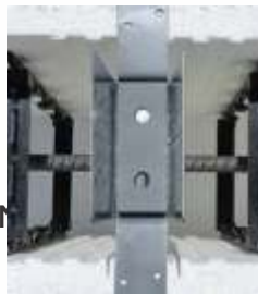
Position BHBCON at truss/rafter mark
